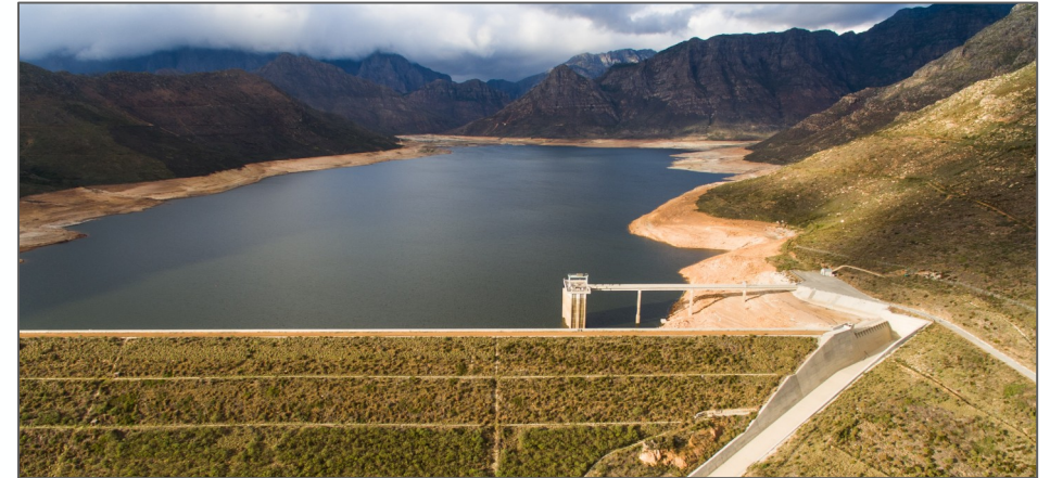
Berg River Dam source: Daniel Saaiman
